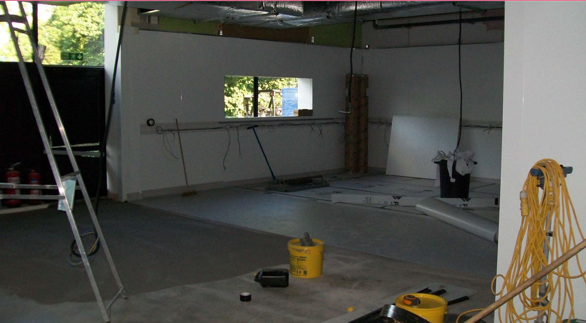
G2- Class 2 lab Electrical and flooring well advanced
